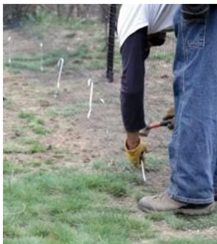
Stakes should be put in a 45 degree angle about every 3-4 feet.
